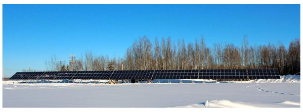
**Figure 1:** Fort Simpson is Northwest Territories Power Corporation's largest diesel-powered community. This 61 kW system (the largest north of 60° in Canada) will help displace 15 000 L of fuel annually and provide up to 8.5 % of the village's minimum power requirements during the summer. (Photo: Skyfire Energy)
