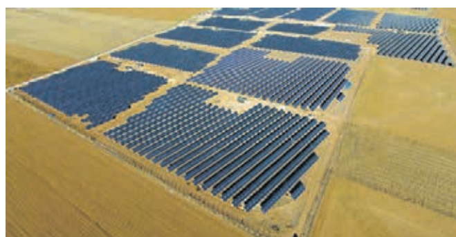
Fig.1 - The largest PV system in Turkey with the installed capacity of 18,5 MW (expected 30,7 GWh annual electricity generation) in Konya (still pending approval for grid connection) [10].
