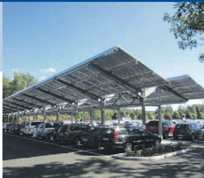
Fig. 3 - First stage on a planned 700 kW PV installation on roofs over a car parking, at Skaraborg Hospital (Photo: Johan Paradis).
