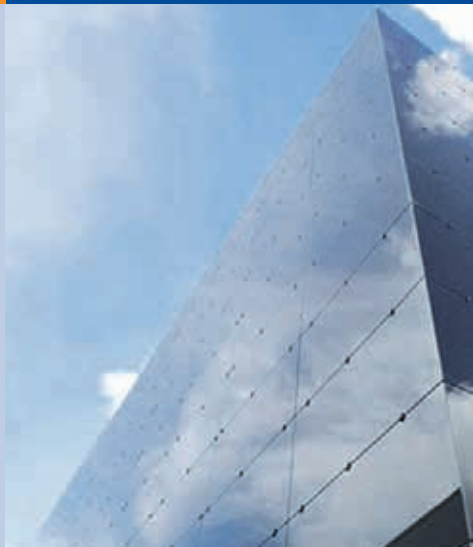
Fig. 3 - BIPV office façade in Spain with a combination of opaque and semi-transparent amorphous silicon photovoltaic glass modules (Photo: © Onyx).
