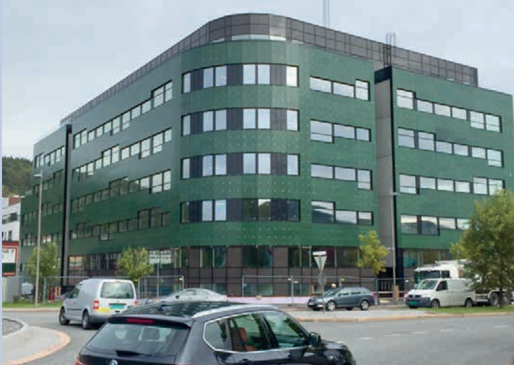
Fig. 1 - 127 kWp of screen-printed glass with integrated PV cells installed in 2015 at Solsmaragden, in Drammen, Norway (Photo: Fusen AS).
