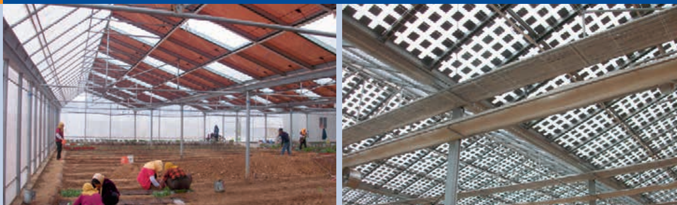
Fig. 3 - PV Integrated with Greenhouses.
