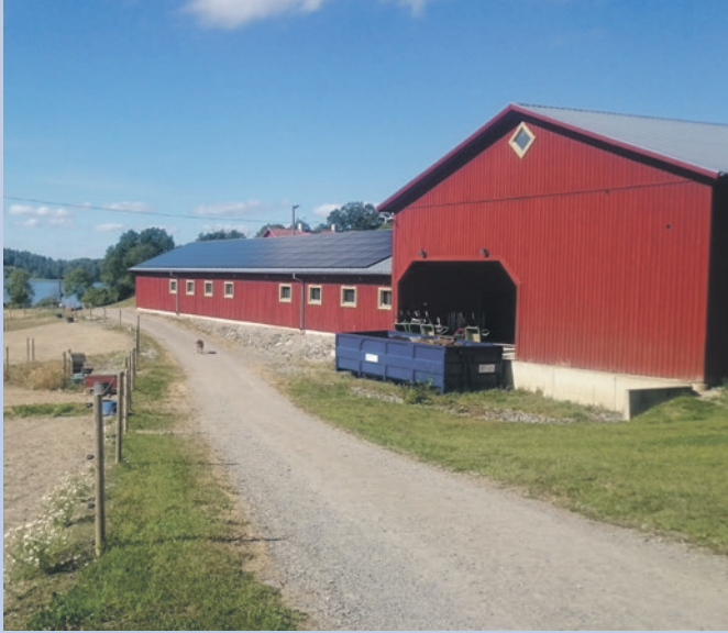
Fig. 1 - 62 kW photovoltaics on barn roof in Bromma Gård, outside of Stockholm (Photo: Solkompaniet).
