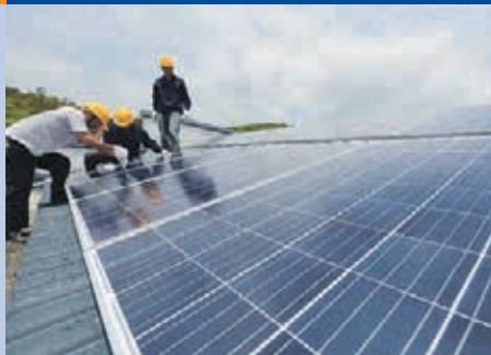
Fig. 4 - Technicians are installing PV system for a rural house in Guzhang county, Jiangxi province.
