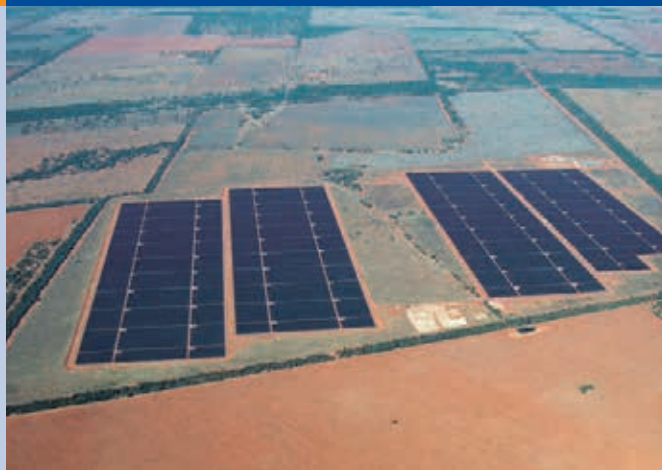
Fig. 2 - The ARENA Solar Flagship Utility Scale Solar Farm, Nyngan NSW. AGL: How we source our energy (Photo: AGL Energy).
