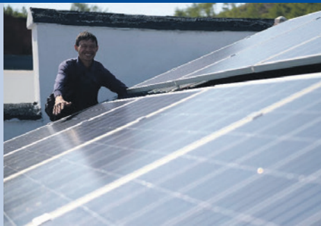
Fig. 5 - A villager is checking PV system on his own house roof.
