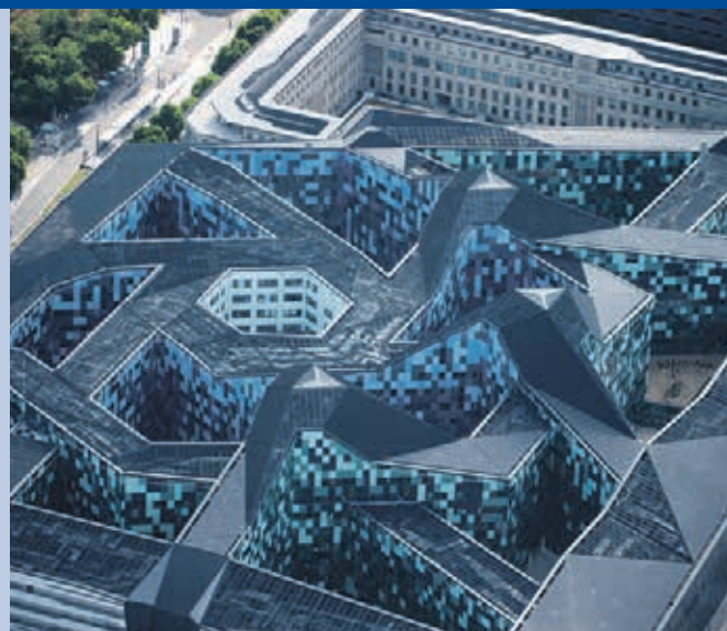
Fig. 2 – 820 kW BIPV rooftop with specially designed zinc coloured c-Si PV modules similar to zinc roofs in Paris (Photo: ANMA, ©R. Nicolas-Nelson/ Armée de l'Air).
