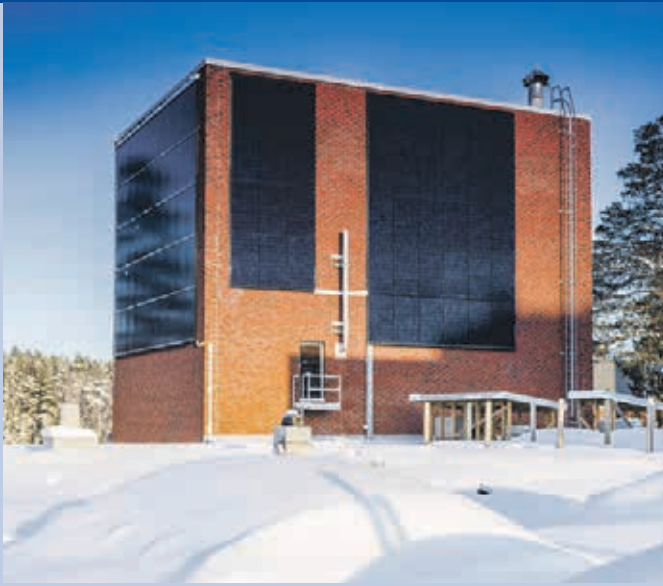
Fig. 1 - Wall-mounted solar PV panels at LUT (Photo: Lappeenranta University of Technology www.lut.fi ).
