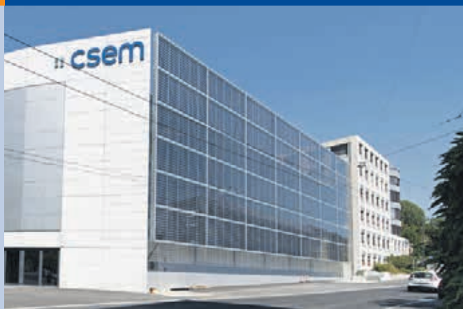
Fig. 4 - New 70 kW PV façade at the CSEM building in Neuchâtel (Photo: CSEM SA).
