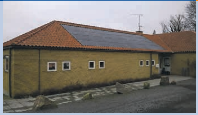
Fig. 4 - Roof integrated PV system by Storløkke holiday centre in Bornholm. A part of the PV Island Bornholm R&D project. Developed by Nielsen EI, Rønne.
