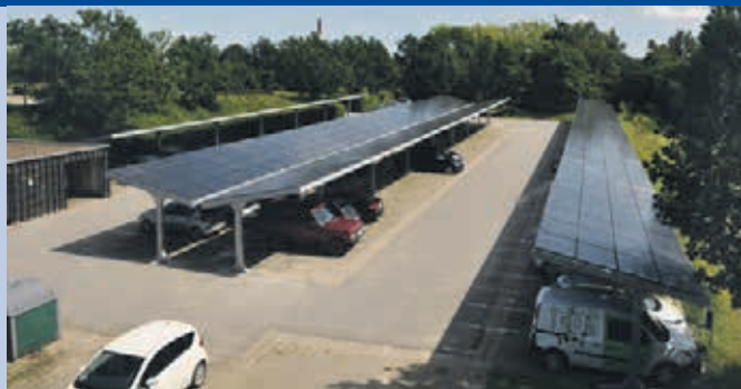
Fig. 1 - Car park with a 152 kWp PV system from the town hall in Fredensborg. Developed by Solar Park.
