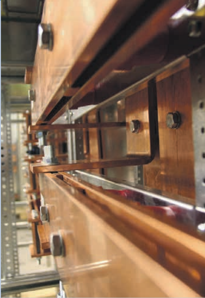
Fig. 1 – Copper busbars.
