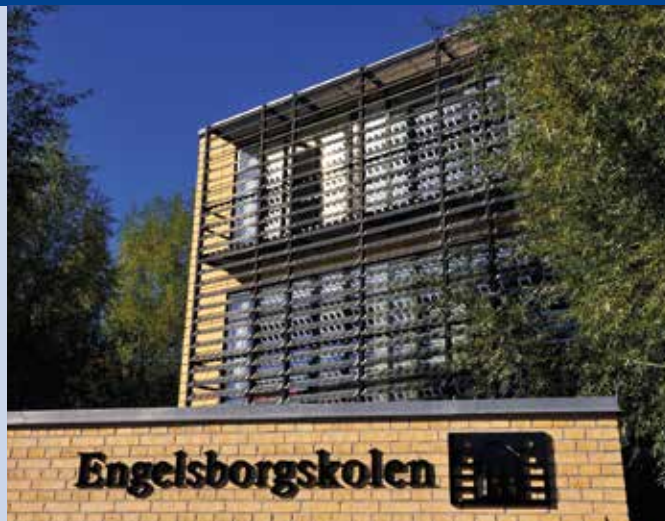
Fig. 1 - 6 kWp mono crystalline PV integrated as shading system in the facade of the school Engelsborgskolen in Copenhagen, developed by Gaia Solar.
