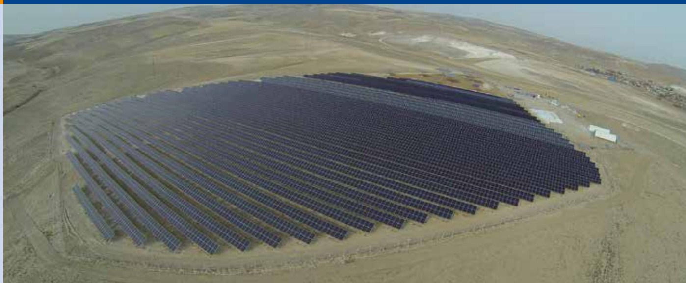
Fig.1 - 1,8 MW grid-connected PV system in Polatli, Ankara.
