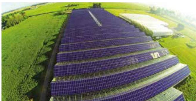
Fig. 1 - At Vine Fresh Produce Project is the largest rooftop installation in Ontario under the FIT program (2,3 MWp). This project is currently the largest system in the world with an Enphase micro-inverter.
