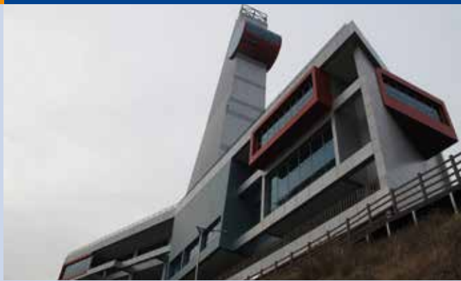
Fig. 3 - 600 kW BIPV system located at Changwon Solar Tower, Gyeongsangnam-do, Korea.
