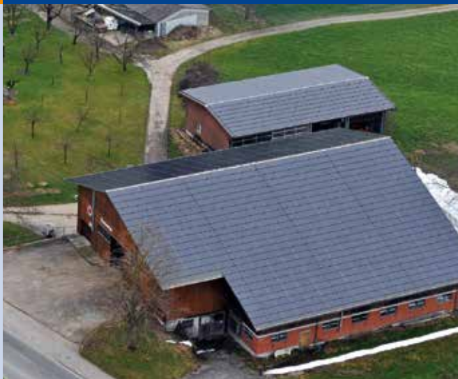
Fig. 2 - Farmhouse in Sempach, Switzerland. 171 kW roof-integrated PV system (Photo: Schürch-Egli AG).
