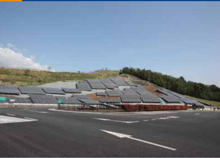
Fig. 2 - Yamada Expressway Service Area (rest area), West Nippon Expressway (NEXCO-West) (Asakura City, Fukuoka Prefecture) Mitsubishi Electric(mc-Si) 1 MW.
