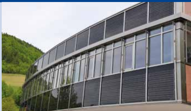
Fig. 1 - Welser Profile Office Building, Ybbsitz, Lower Austria. BIPV (Mcsi) Facade, RP-Technik ISO 60 hermetic, stainless steel (Photo: Welser Profile).
