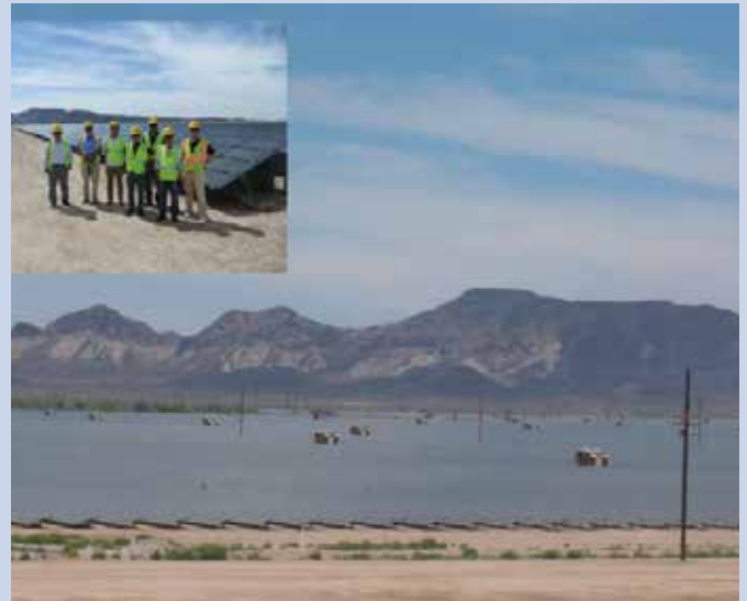
Fig. 2 - Agua Caliente PV power plant- technical visit at the 29 th Task 8 meeting in Arizona, USA, in June 2013.
