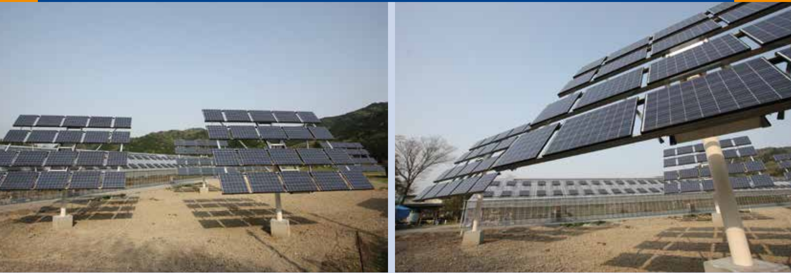
Fig. 3 - Fujipream's Experiment Farmland (Himeji City, Hyogo Prefecture) Tracking PV Systems: 30 kW, Greenhouse: 20 kW Fujipream (mc-Si).
