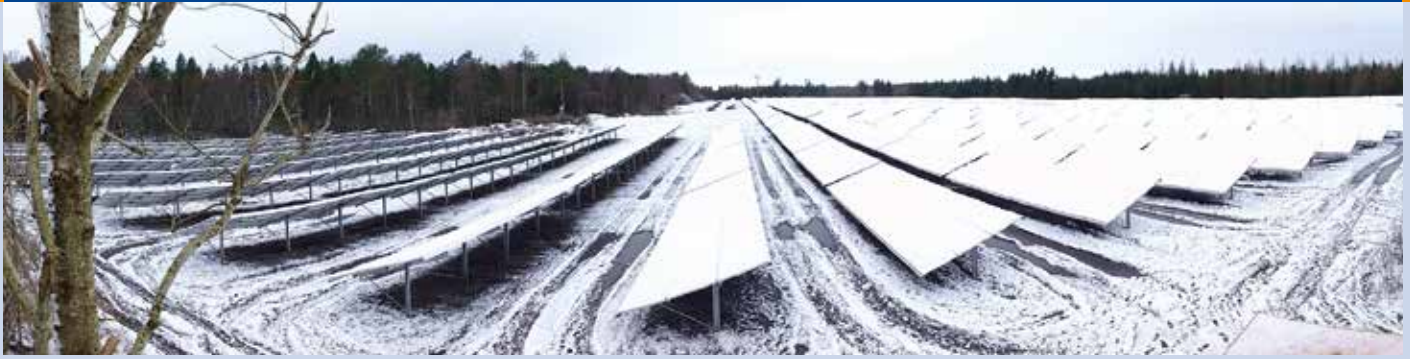
Fig. 3 - 2,4 MW ground mounted system divided into 5 strings. The system is developed by Sveigaard Ltd. and located near by the city of Herning.
