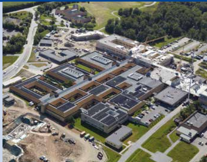
Fig. 2 - 306 kWp PV system on the roofs of the hospital, Sygehus Sønderjylland, in Danish city Aabenraa. All hospitals in this region are equipped with PV systems.
