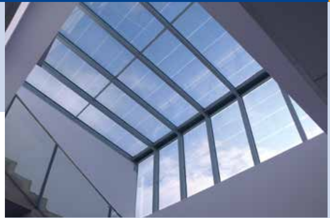
Fig.6 - BIPV installation in the "Lucia" Building, Miguel Delibes Campus of Valladolid University (2013) (Source: ONYX SOLAR).
