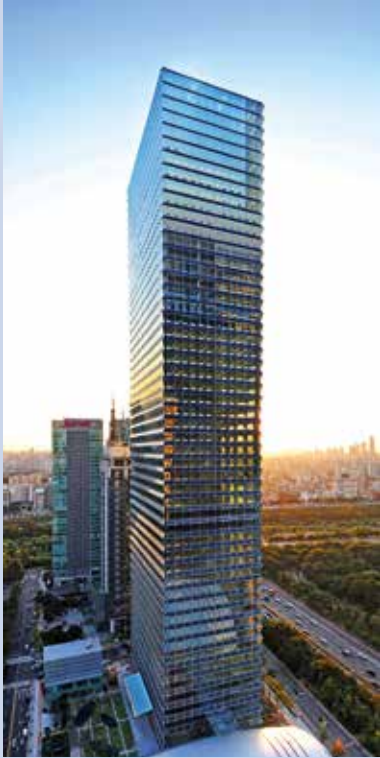
Fig. 1 - 728 kW BIPV system located at Federation of Korean Industries Head Office Building, Seoul, Korea.
