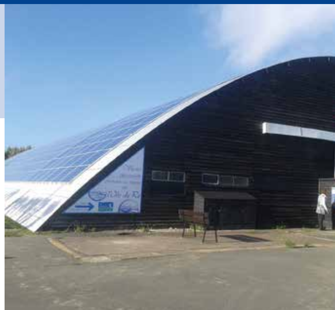
Fig. 3 – 100 kW installed on the roof of the building of the Cooperative processing and packaging sea salt in the Île-de-Ré (Photo: Solarsit).
