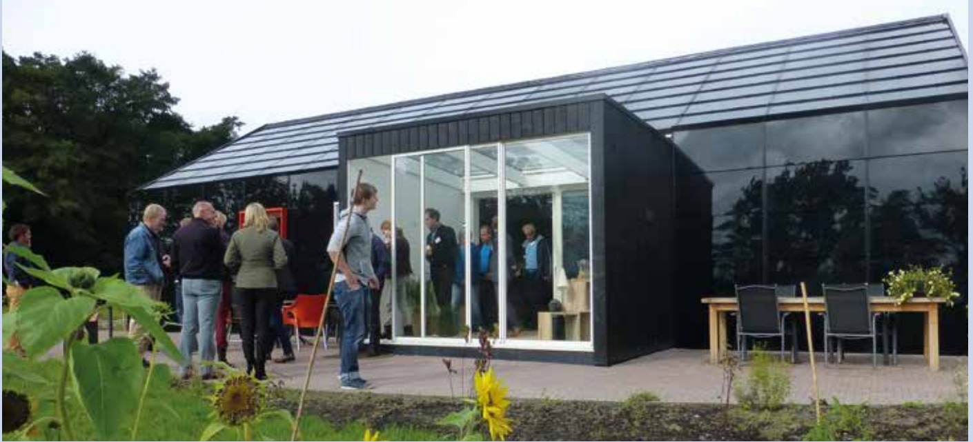
Fig. 1 - Private house design by owner, M. de Graaf with 125 m 2 of solar panels (Photo: RVO).
