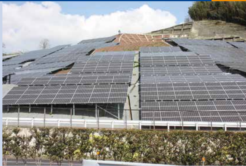
Fig. 2 - Yamada Expressway Service Area (rest area), West Nippon Expressway (NEXCO-West) (Asakura City, Fukuoka Prefecture) Mitsubishi Electric(mc-Si) 1 MW.
