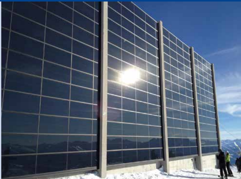
Fig. 5 - Ski station, Laax, Switzerland. 21 kW PV-façade with CIS modules (Photo: Solarmarkt GmbH).
