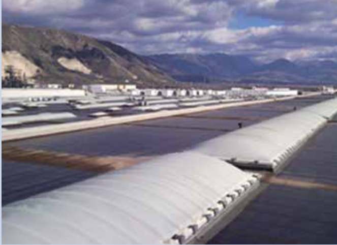
Fig. 1 - 1 544 kWp PV plant at Nola (NA), using General Solar Flexible Modules (thin film on flexible support) (Photo: GSE, Gestore del Sistema Elettrico).
