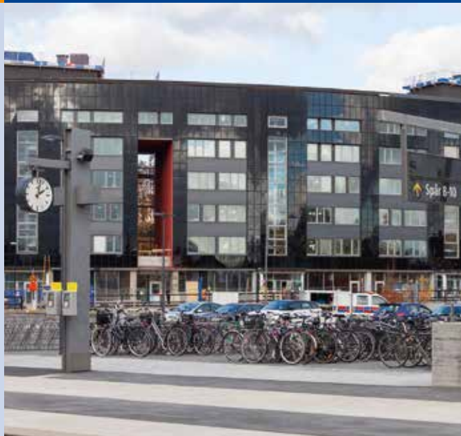
Fig. 3 - Façade integrated thin film modules in the city of Uppsala (Photo: Thomas Zaar, White Arkitekter AB).
