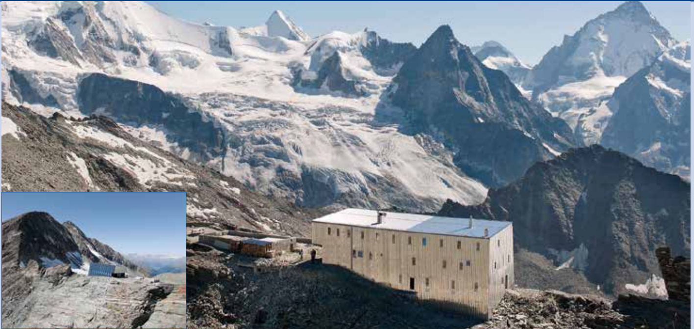
Fig. 1 - Cabane Tracuit. Off-grid alpine hut at 3 256 m. 11 kW PV-façade together with 1 500 Ah battery storage (Photo: Studer Innotec SA).
