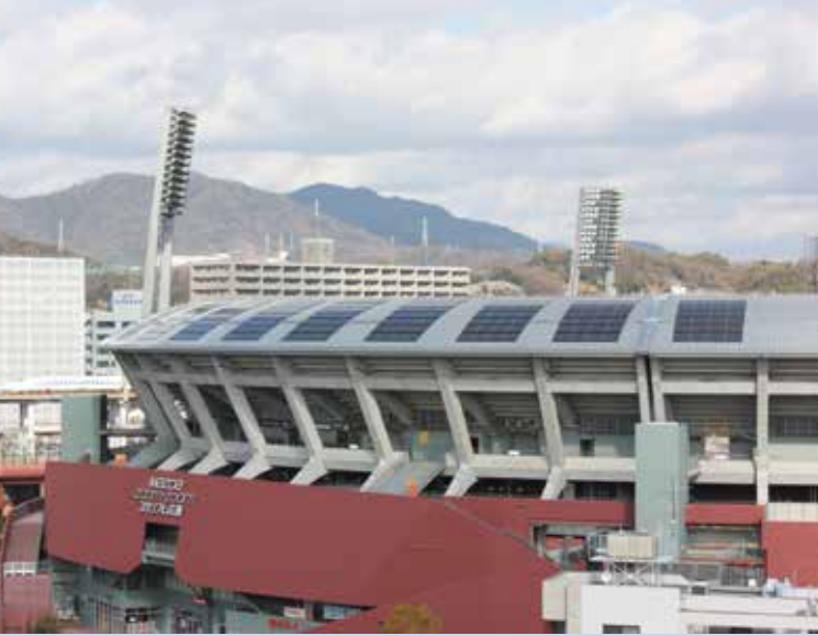
Fig. 1 - MAZDA Zoom-Zoom Stadium Hiroshima (Hiroshima City, Hiroshima Prefecture) Kyocera (mc-Si) 100 kW.
