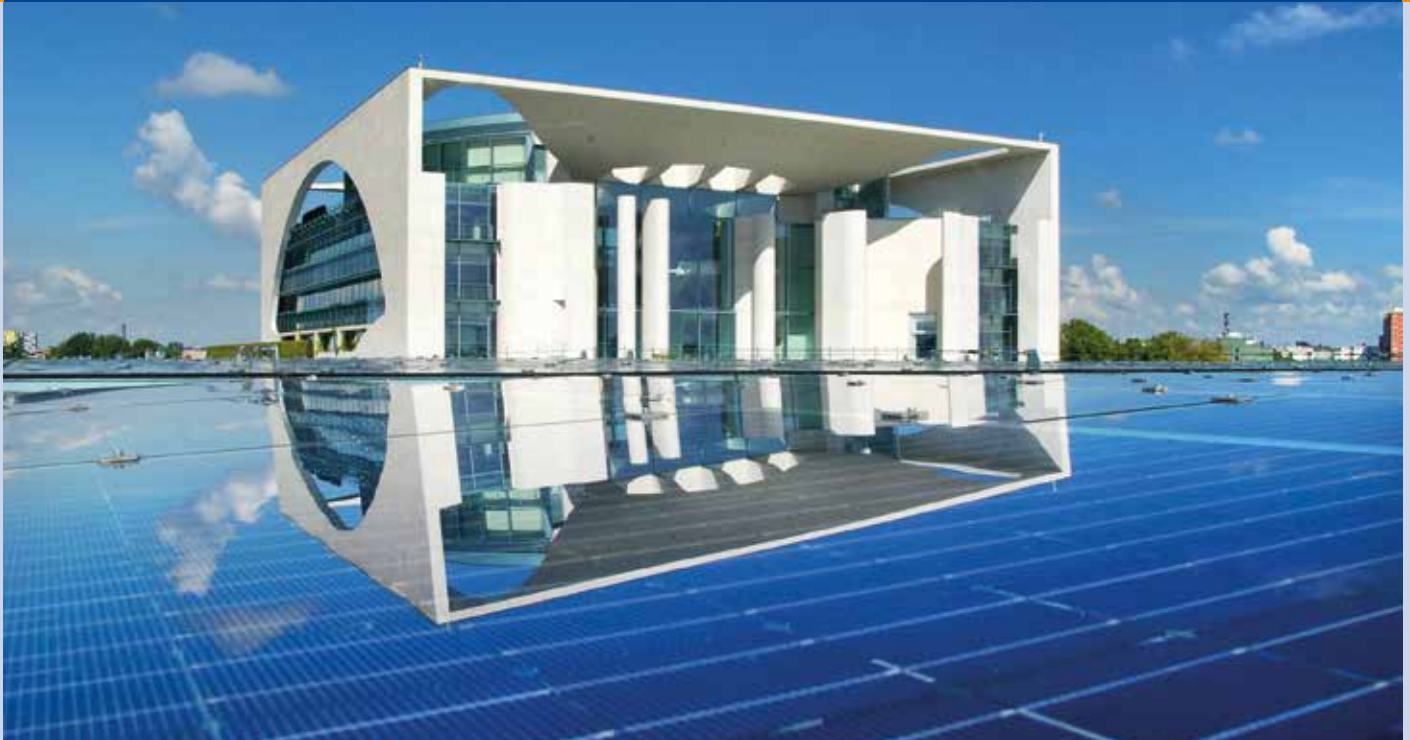
Fig. 2 – 150 kWp photovoltaic system on the rooftop of the German Chancellery (Photo: BSW-Solar/Langrock).
