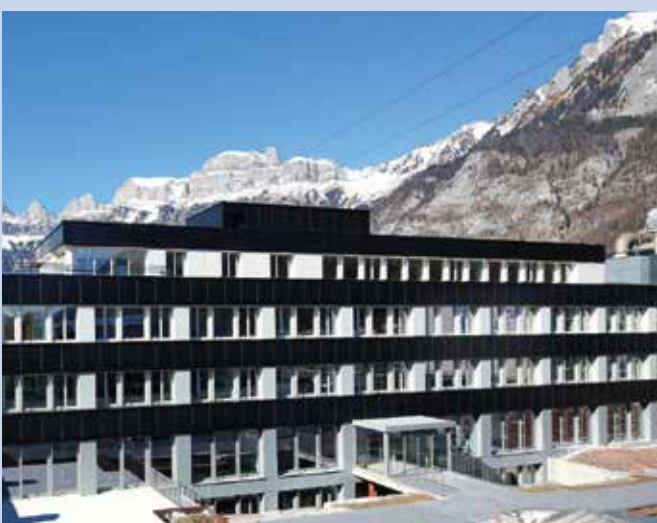
Fig. 3 - Office building from Flumroc Ltd. PV-façade and on-roof system, 128 kW in total (Photo: Viridén + Partner AG).
