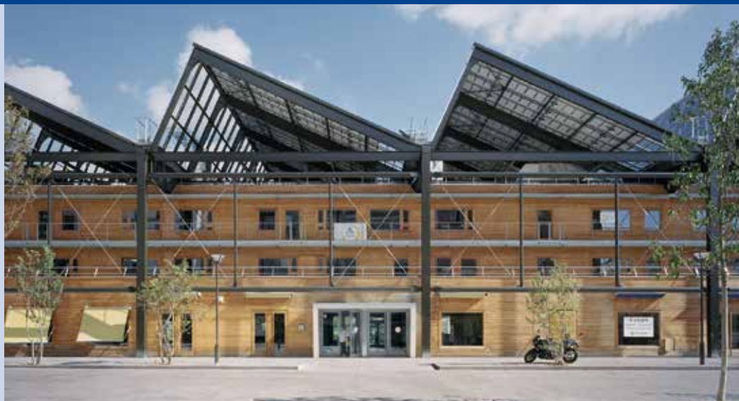
Fig. 2 – Halle Pajol, low energy building, 500 kW on a reclaimed railway facility in Paris (Photo: Jourda Architect).
