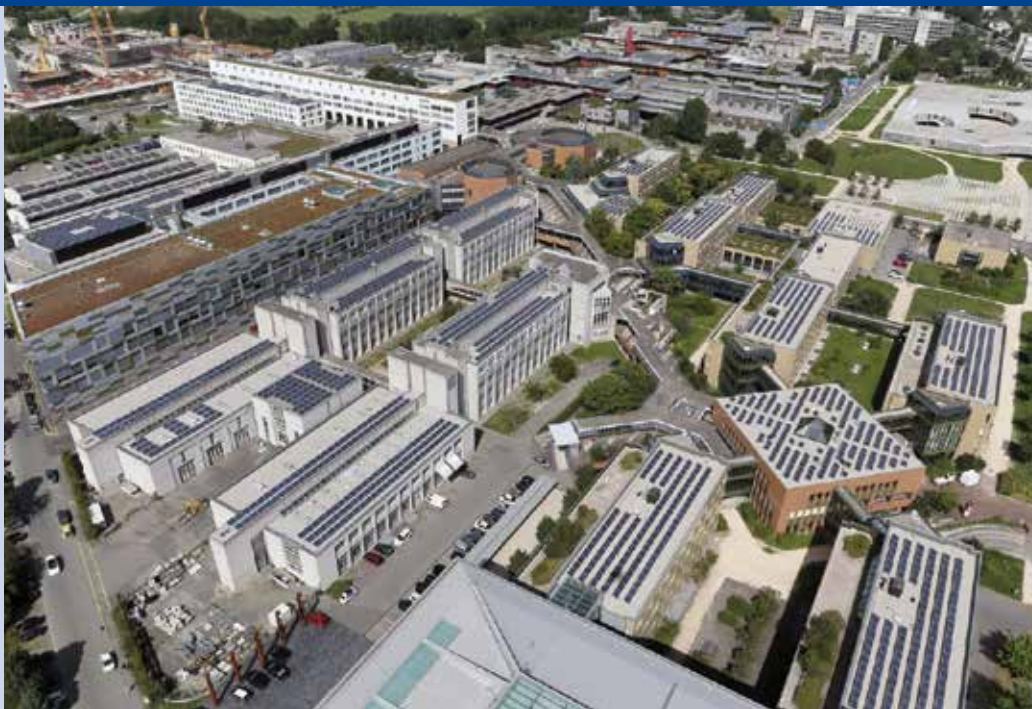
Fig. 6 - EPFL Campus, Lausanne, Switzerland. 2 MW on-roof PV systems featuring different kinds of technologies (Photo: Romande Energie).
