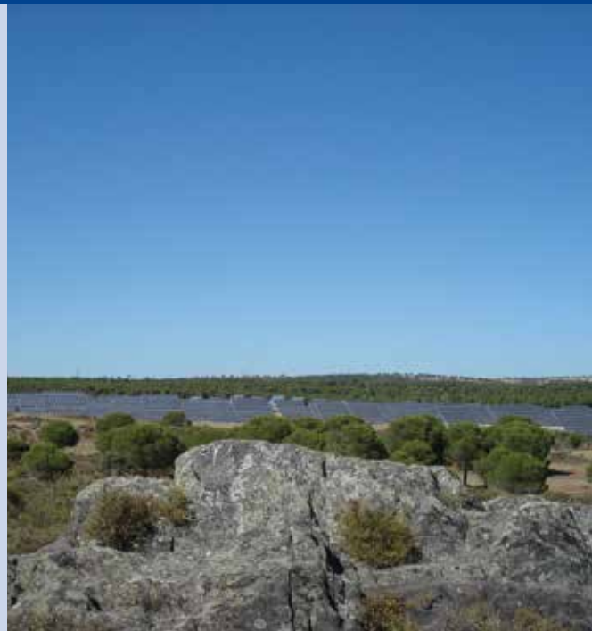
Fig. 2 - 46 MWp PV plant in Amareleja, Portugal.
