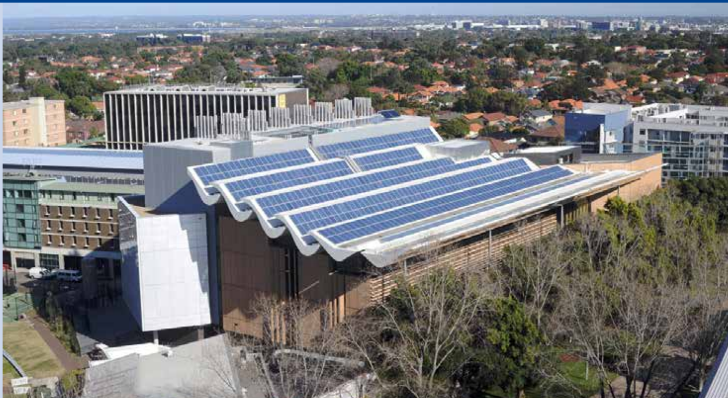
Fig. 1 - 120 kW PV array on the 6 Star Tyree Energy Technologies Building, UNSW Australia (Photo: UNSW).
