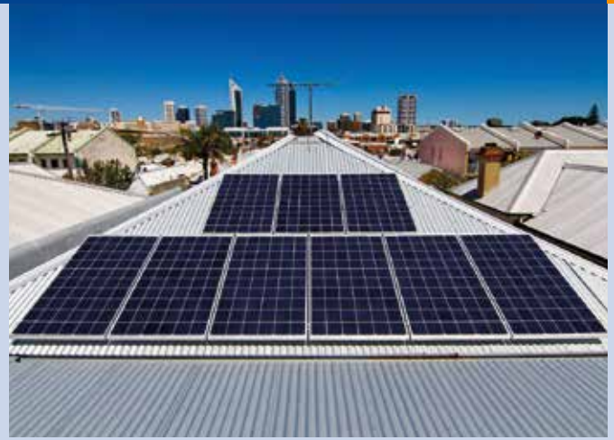
Fig. 3 - 2,1 kW residential array in Perth, using Hanwha Q.Cell's Q.Pro-G2 modules (Photo: Hanwha Q.Cells Australia).
