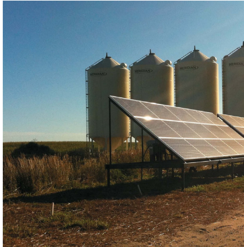
10kW system installed at an irrigation pivot and grain drying facility near Picture Butte, AB. Photo courtesy Sustainable Energy Technologies.
