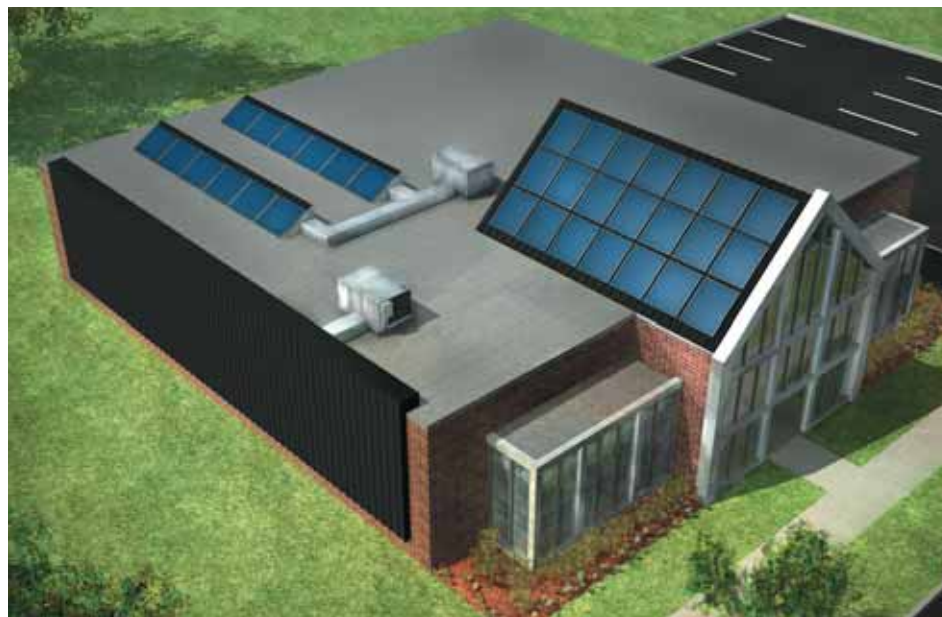
Concept drawing that shows the combination PV/thermal technology. Photo courtesy of Conservall Engineering, Inc.
