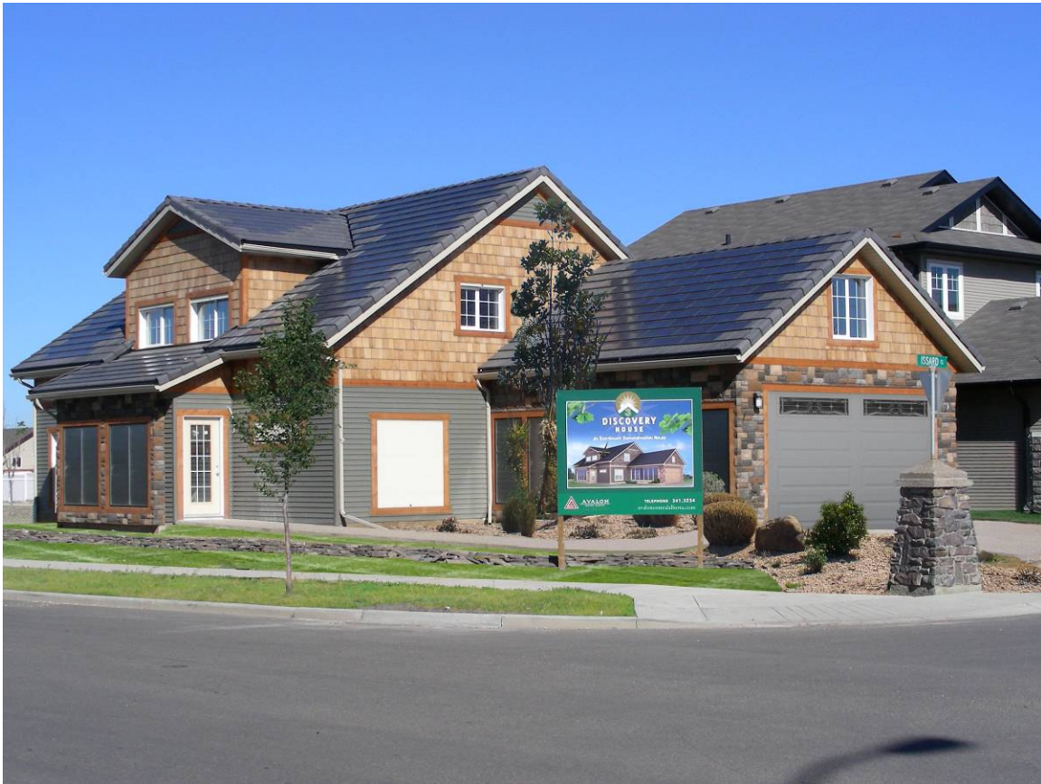
Figure 1: The Avalon Discovery EQUilibrium™ House, Red Deer, Alberta, Canada. (Photo credit: Avalon Master Builder)
