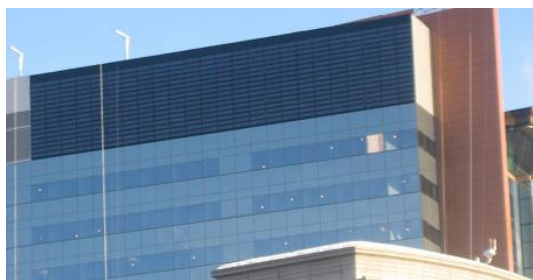
Figure 4: Schematic of the he combined solar PV – Thermal installation at the JMSB. (Credit: B. O'Neill, Canadian Solar Buildings Research Network)
