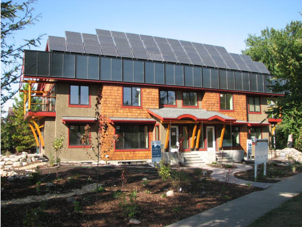
Figure 2: The Riverdale Net Zero Energy duplex, Edmonton, Alberta, Canada. (Photo credit: CMHC)
