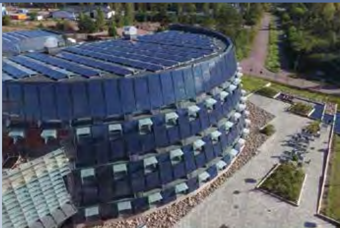
Fig. 1 - The head office of PAF Oy in Mariehamn in Åland (Photo: Naps Solar Systems Oy).
