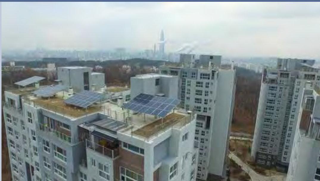
Fig. 3 - 142 kW roof mounted PV system installed by PV rental programme, Seoul, Korea.
