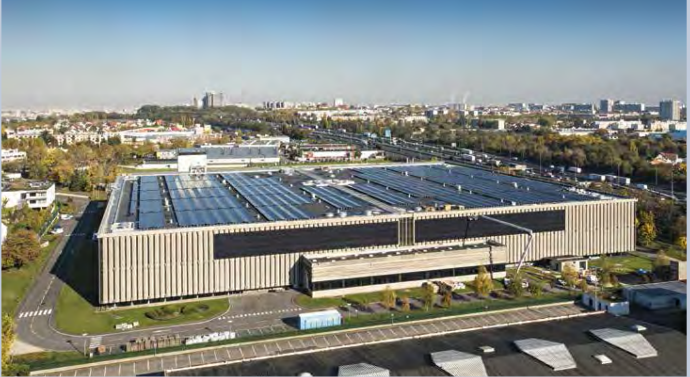
Fig. 1 - 1,8 MW on Eaux de Paris reservoirs at L'Hay-les-Roses that supply the city of Paris with drinking water (Photo: Studio VU - SOPREMA Entreprises).
