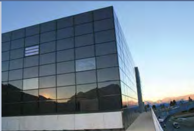
Fig. 1 - Penken Cable Car Station, Tyrol (Photo: © ATB Becker).
