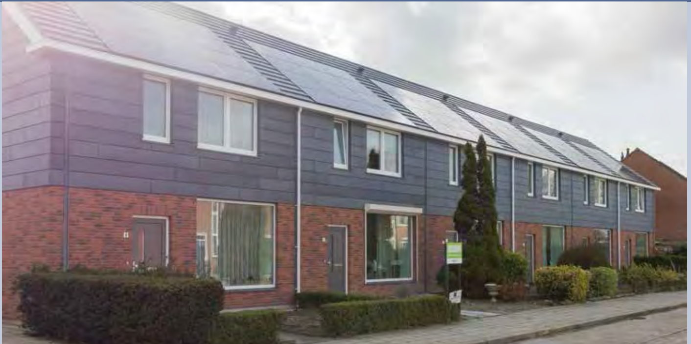
Fig. 1 - Renovation social housing in Goes, Province Zeeland, courtesy of Marsaki (Photo: Marsaki & RWS partner in wonen).
