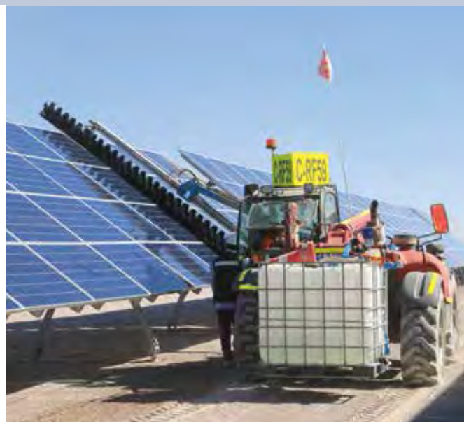
Fig. 5 - PV Cleaning System. 160 MW Finis Terrae PV Plant (ENEL Green Power) located at María Elena, Antofagasta Region, Chile.
