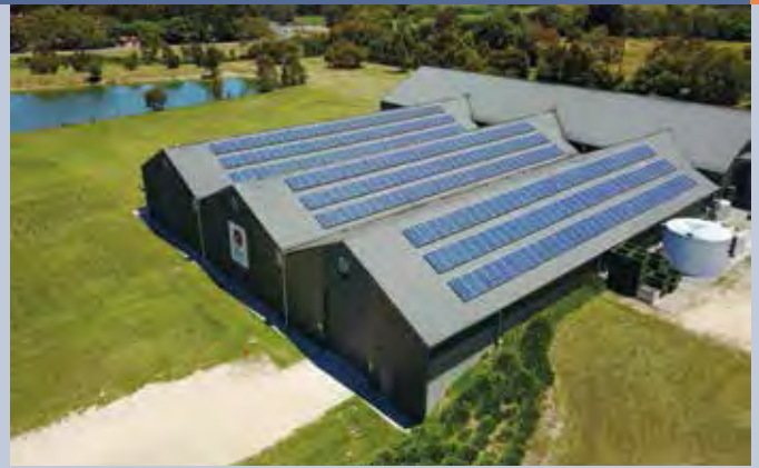
Fig. 4 - Wicks Winery Estate. Woodside, South Australia. 80 kW system sold and installed by Venergy Australia (Photo: Matt Wilkins).
