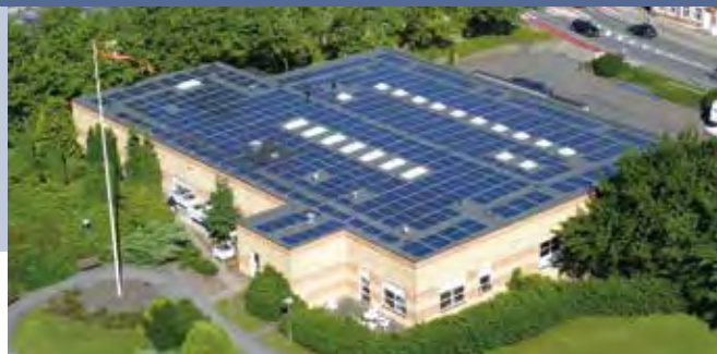
Fig. 2 - PV Solar Systems at the Regional Hospital in Viborg: A total of 280 kWh has been installed on 5 roof and area covering app. 10 % of the annual consumption at the hospital (Photo: Kenergy, Kenn H. B. Frederiksen).
