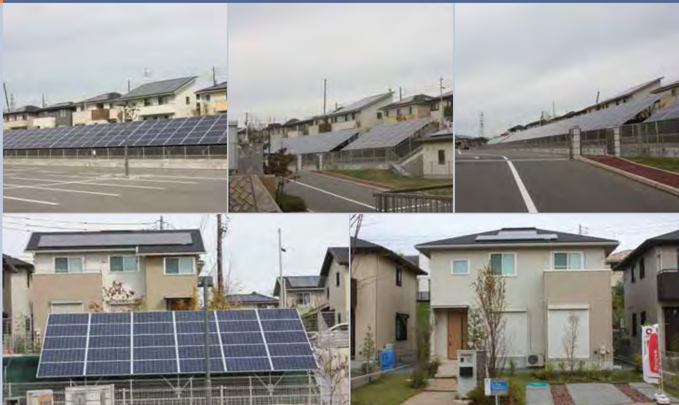
Fig. 2 - Smart Town with PV systems installed on all houses as standard (Sma x Eco Town Hidamari no Oka) (Kuwana City, Mie Prefecture). Houses: 66 residential PV systems (ca. 330 kW in total), Ground-mounted PV system: 100 kW, Multicrystalline silicon PV modules (by Sharp).
