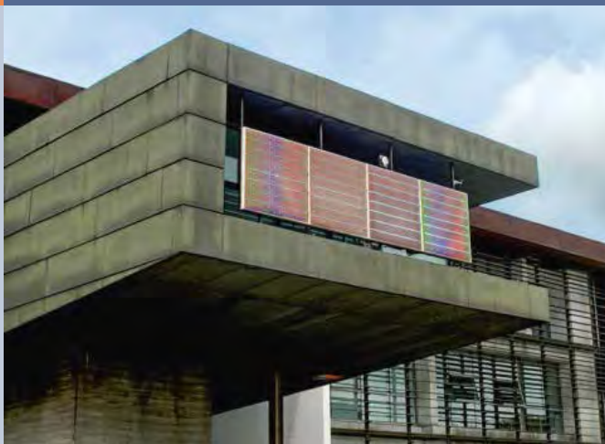
Fig. 4 – Demonstrator installed in ITMA building out of BIPV elements (transparent PV and LED integrated) developed in the ETFE-MFM project.
