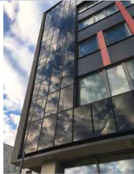
Fig. 1 - Task 15's visit to the Frodeparken Building, Uppsala, Sweden.
