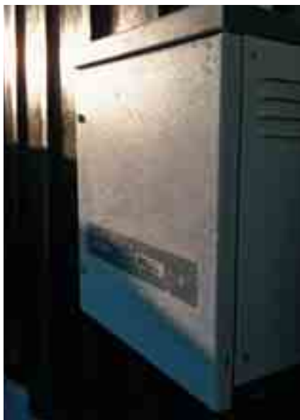
SUNERGY Inverter for the Enmax-Paralex Demonstration 10kW rooftop system at Strathcona-Tweedsmuir School, Okotoks, Alberta
