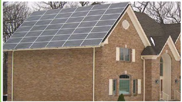
Typical retrofit. Note: No clearances along edges
