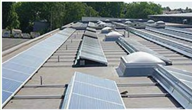
Flat roof with ballasted or attached installation
