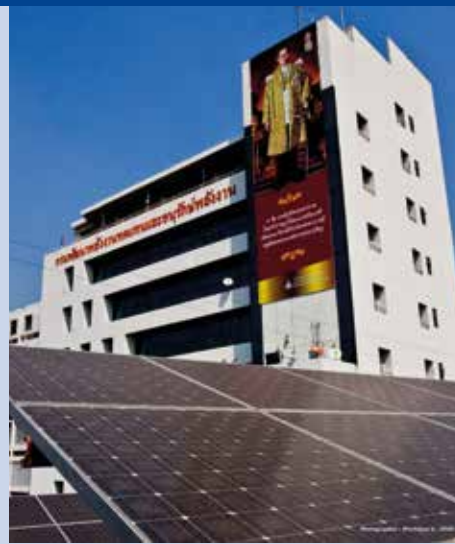
Fig. 3 - Solar PV Rooftop System 5 kWp at Department of Alternative Energy Development and Efficiency, Bangkok, Thailand.
