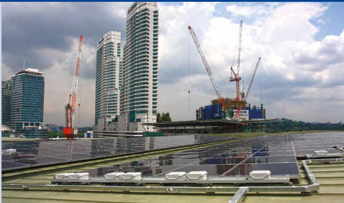
Fig. 1 - Lot E, KL Sentral (168kWp), Platinum rated "Green Building" (Photo: Pekat Teknologi Sdn Bhd).
