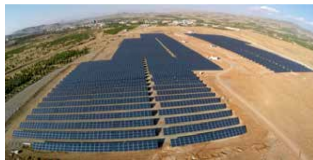
Fig. 1 - The largest PV system in Turkey with the installed capacity of 5,3 MW in Malatya.
