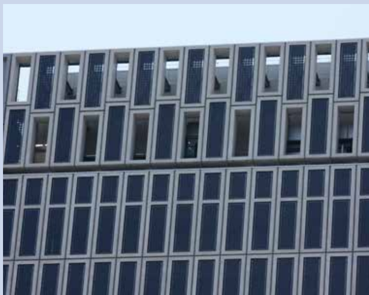
Fig. 3 - Shimizu Corporation headquarters building (Kyobashi, Chuo Ward, Tokyo). 150 kW Multicrystalline silicon PV module. 368 modules: 110 kW (by Sharp). Light-through thin-film silicon PV module 594 modules: 40 kW (by Sharp).
