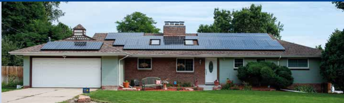
Fig. 1 - A residential home retrofitted with photovoltaic (PV) panels in Lakewood, CO (Photo: Dennis Schroeder / NREL).
