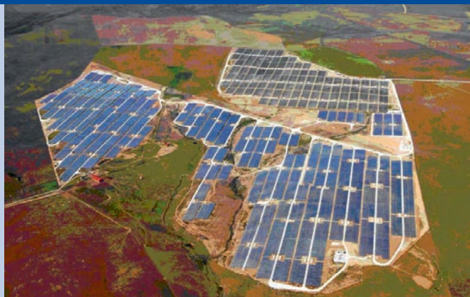
Fig. 1 - PV plant from ATERSA, 30MW, one axis horizontal, c-Si technology in Cáceres, Spain.
