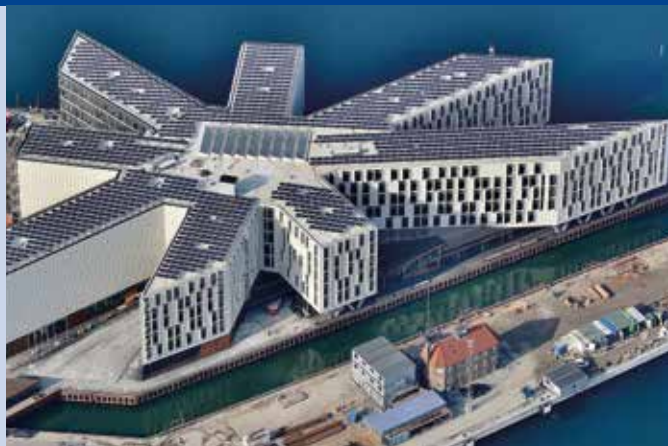
Fig. 1 - The United Nations City Building, situated in the Port of Copenhagen, is one of the most prestigious new buildings in the Danish capital. It is not only an architectural star, but also an environmental one. One of the installations is a special designed 348 kWp PV-plant on the white rooftop. The special design, using a PV-plant as an architectural finesse, won the PV-company, SolarElements, a prize at the Intersolar in Munich 2014.
