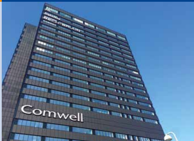
Fig. 2 - Aarhus City Tower. The system is produced by the Danish company, Racell SAPHIRE, and integrated as a 1 800 m 2 BIPV with a maximum power of 250 kWp. The building is fulfilling the energy performance building directive 2015. In the design phase, the focus was on architectural design, façade integration and energy production.
