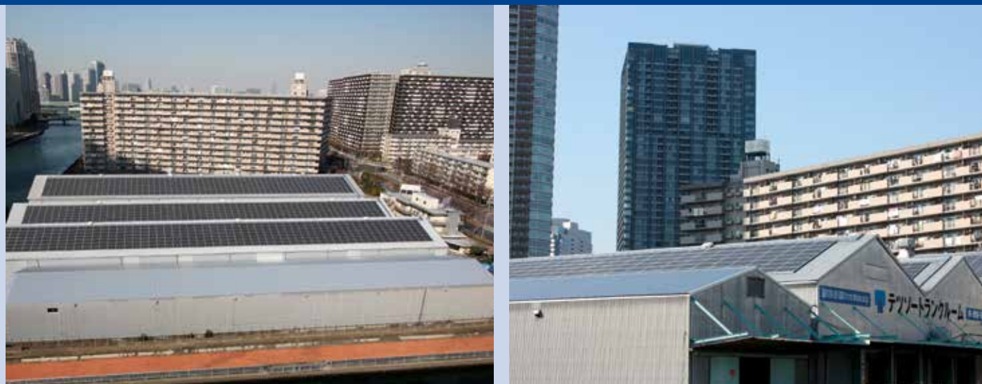
Fig. 1 - TETSUSO's Rental Storage Facilities (Koto Ward, Tokyo). Single-crystalline silicon PV module (by Mitsubishi Electric) 2,9 MW.
