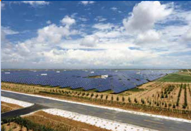
Fig. 3 – 520 MW Longyangxia Hydropower PV station, Gonghe, Qinghai, China (Photo: Yellow River Hydropower Company).
