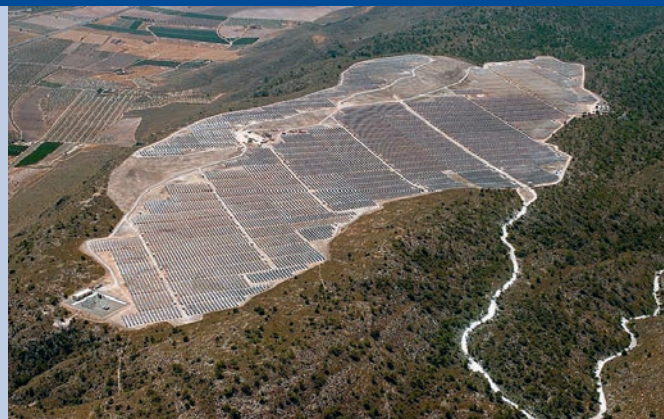
Fig. 3 - PV plant built by ATERSA, 20MW, one axis horizontal, c-Si technology, in Jumilla, Spain.
