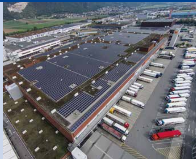
Fig. 7 - 32 000 m 2 PV system with 5,2 MWp, producing 6,8 GWh per year, Migros, Neuendorf (Photo: © NET Ltd. /DanielForster.com).
