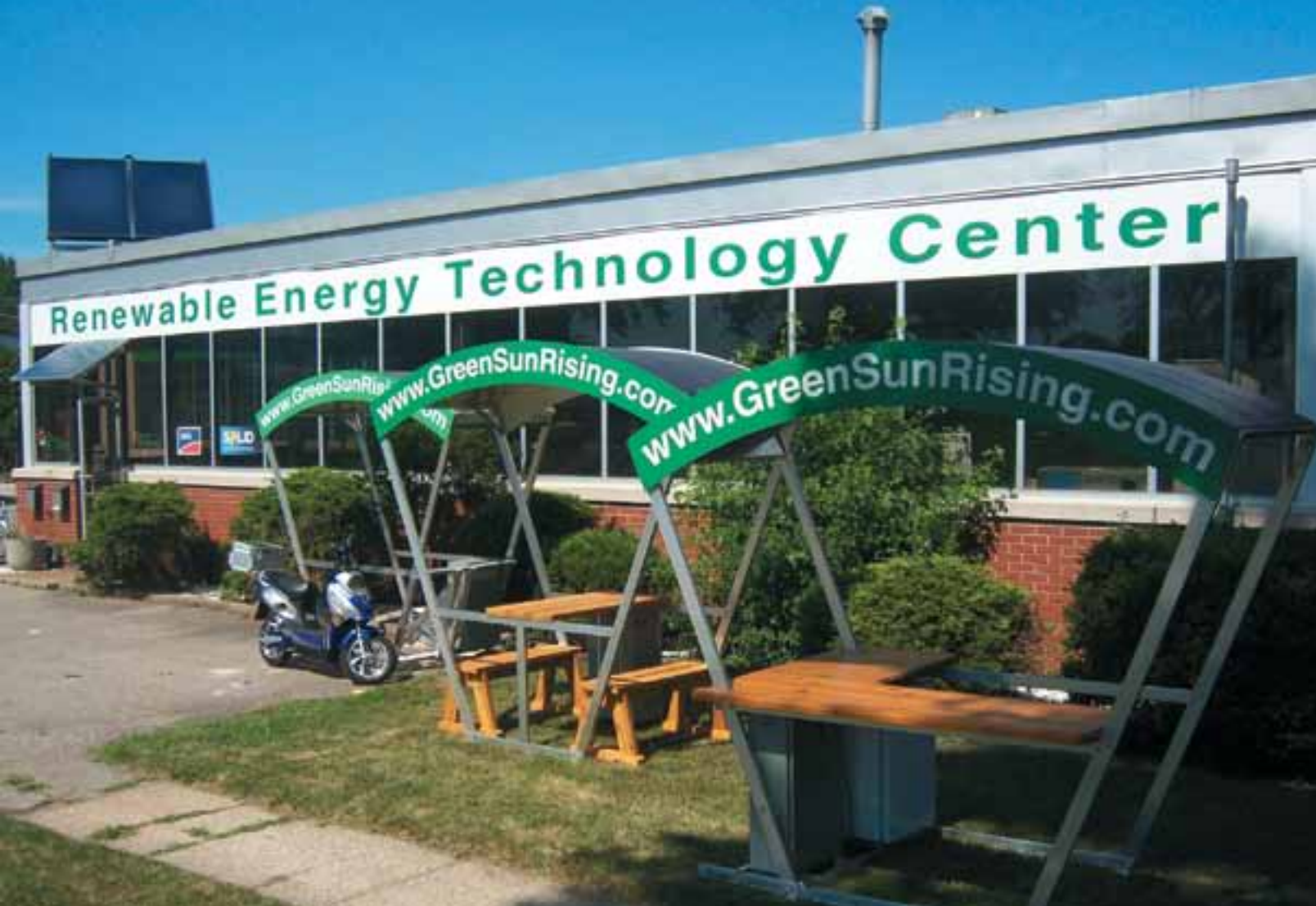
Three-off grid solar systems at the Renewable Energy Technology Center in Windsor. Photo courtesy of Green Sun Rising.
