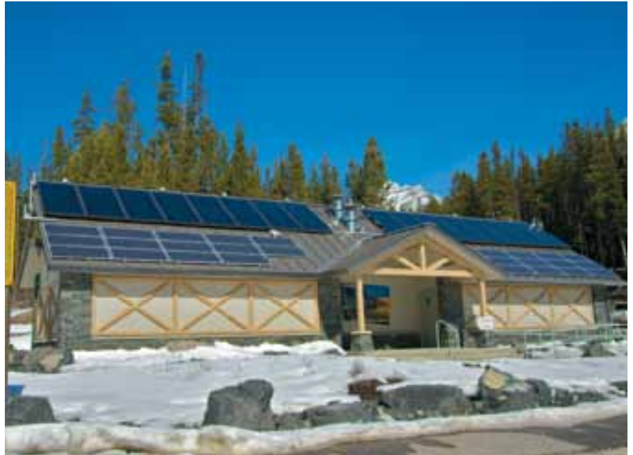
Photo courtesy of SkyFire Energy.
